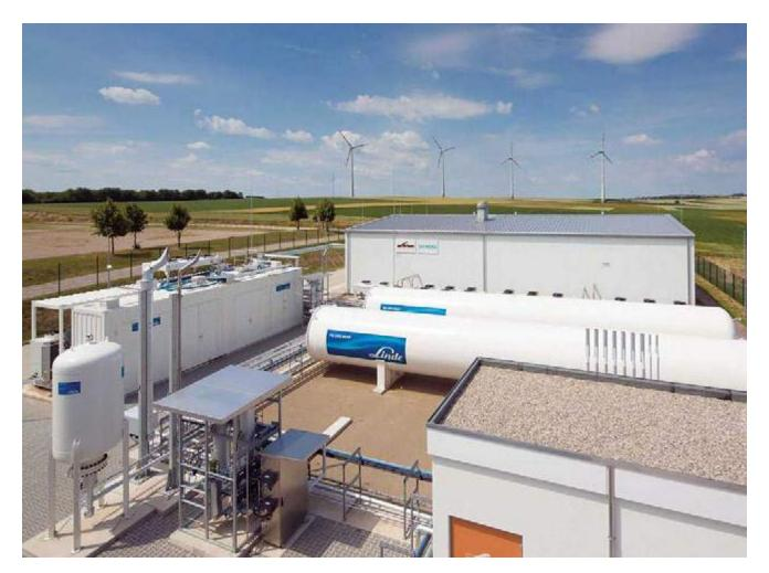
"Energiepark Mainz" located in Mainz, Germany, is connected to an 8 MW wind farm. Three electrolysis units can produce 1000 Nm<sup>3</sup> hydrogen per hour (89.8 kg/h). Photo credit: Stadtwerke Mainz AG
